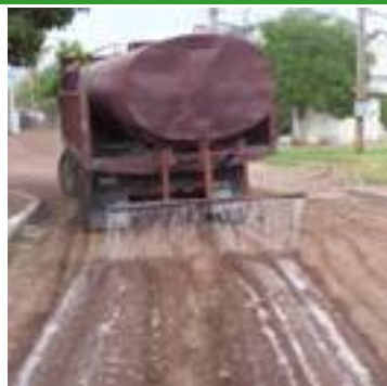
Step 2: Apply Enzyme with Water Truck
